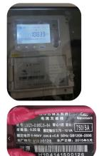
New Plant 2: 91.97 x 100 = 9,197 kWh (the transformer ratio for the new Plant 2 is 500/5 = 100)
