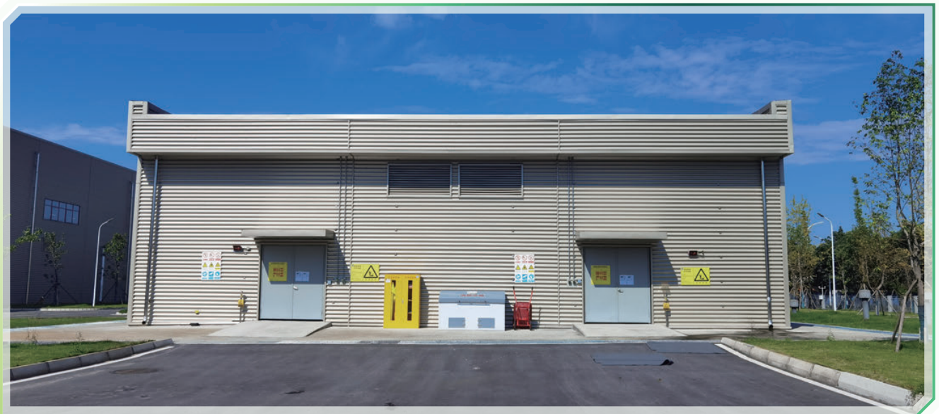
Hazardous waste storage warehouse
