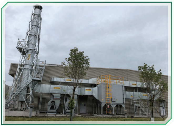
Hazardous waste facilities for waste gas collection and purification in Chengdu plant
