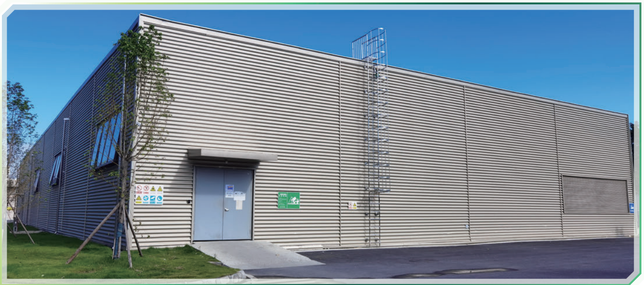
Non-hazardous waste resource recycling warehouse
